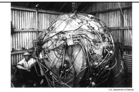
Exposed wiring of "The Gadget," the nuclear device that exploded as part of Trinity. At the time of this photo, the device was being prepared for its detonation.
